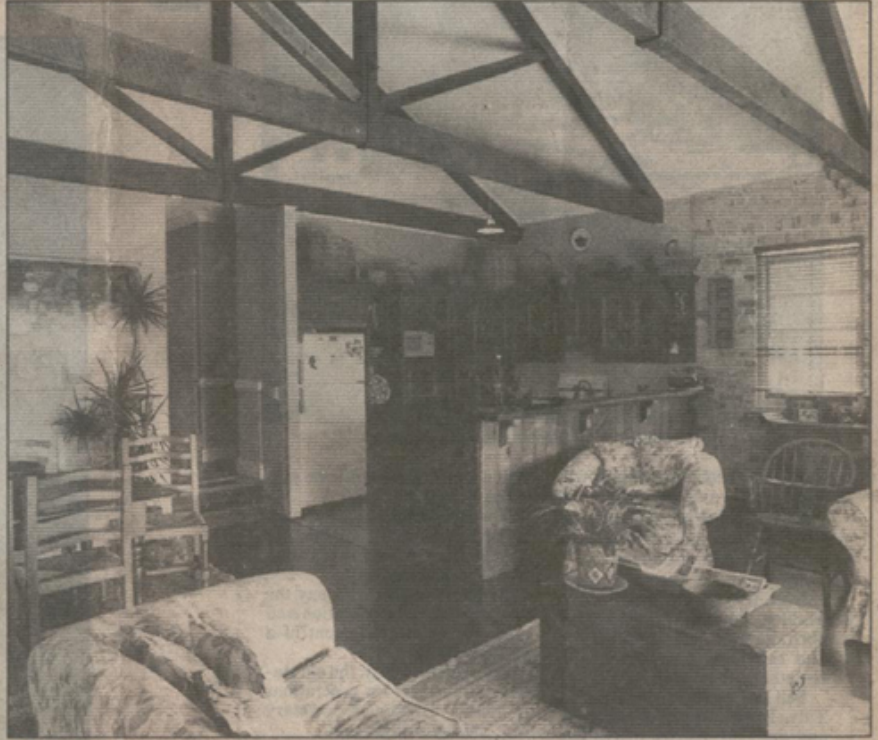
Living room uses second-hand bricks and overhead trusses from an old railway workshop
